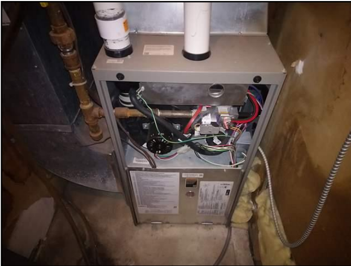
High-efficiency gas furnace
